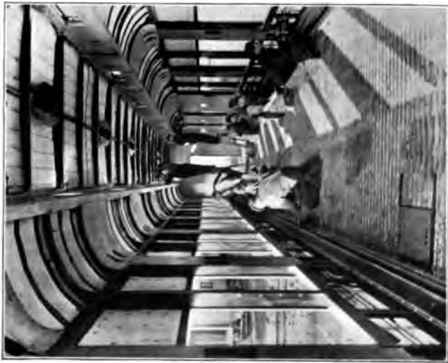
Fitting the car with steam pipes and electric conduits
